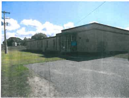
Wastewater Treatment Plant
